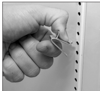
Fig. 1. Installing top tab of shelf clip.
